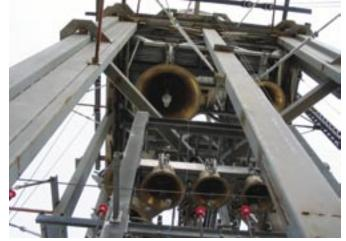
The structural steel framing supports a 50,000 lb, 49-bell carillon in addition to a 14,000 lb pre-manufactured steeple.
